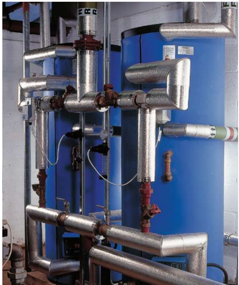
Modular installation of Powerstock calorifiers
