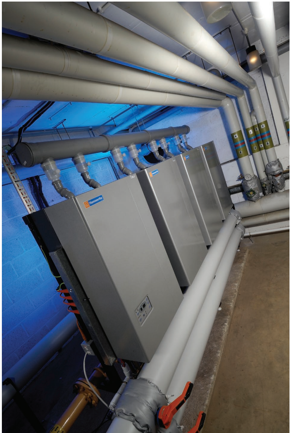
Milborne condensing boilers provide impressive efficiencies
