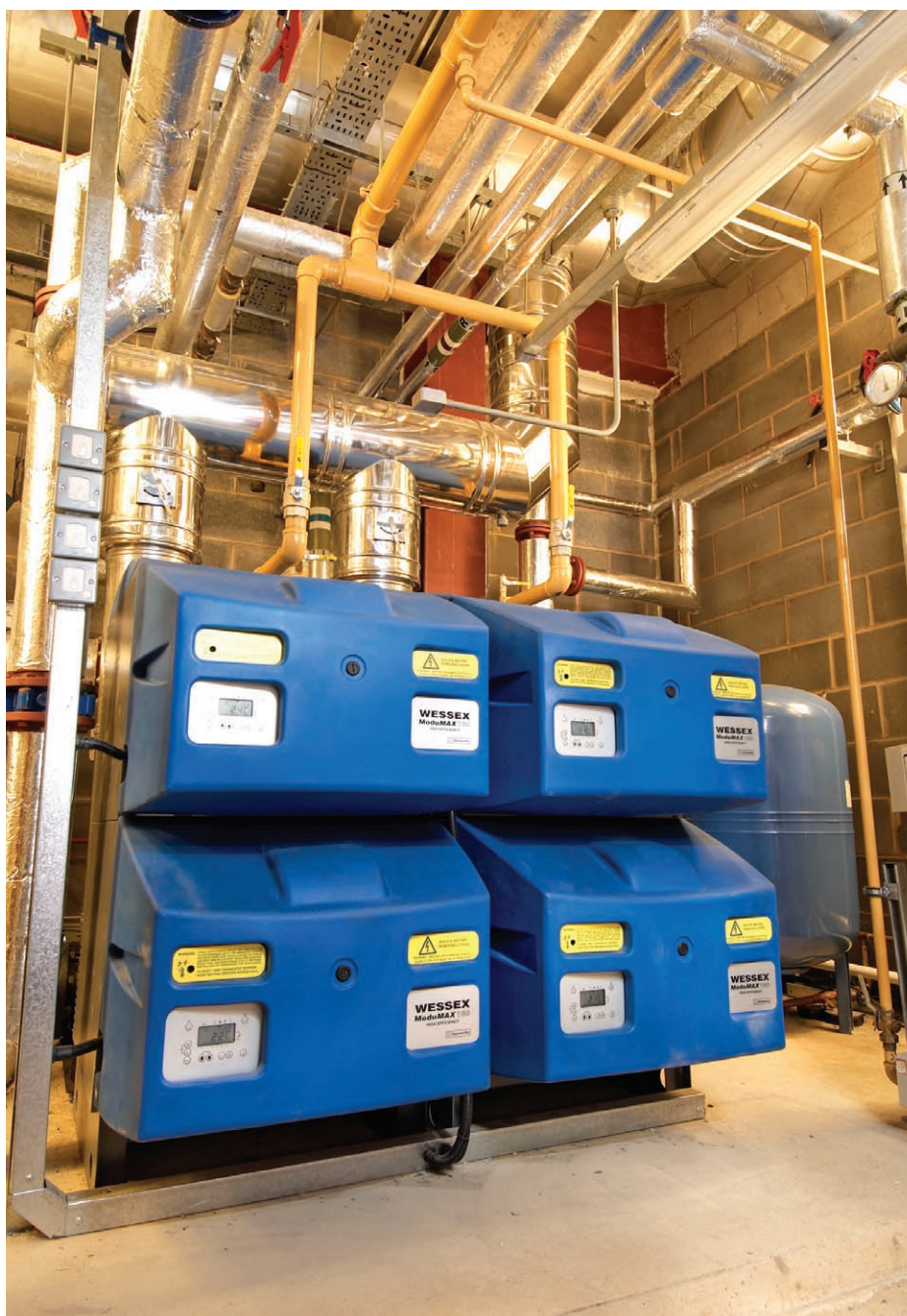
Wessex ModuMax boilers providing 640kW in just 1.5 square metres of floor space
