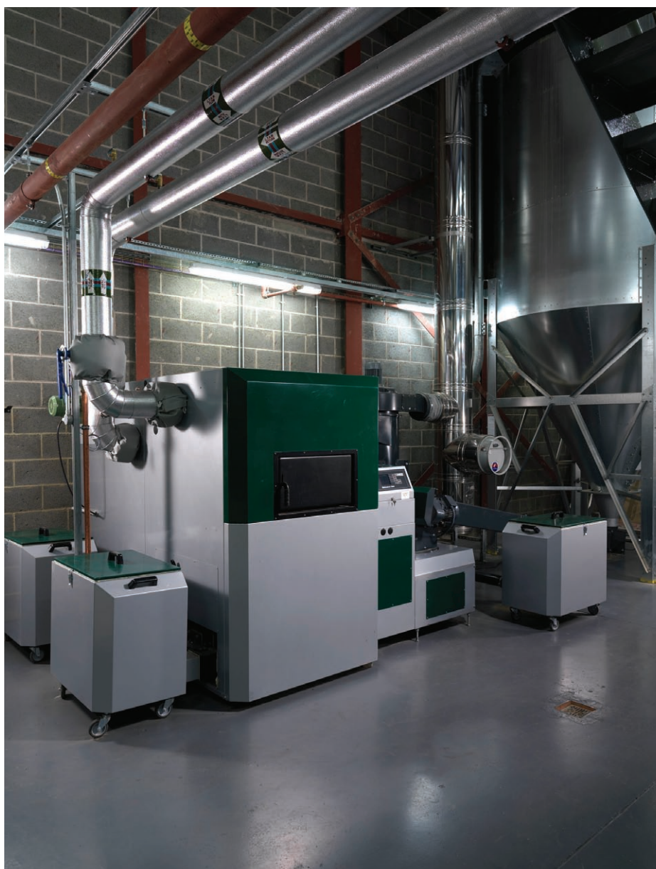
The Hamworthy Biomass system with fuel hopper, flue cyclone and integrated controller
