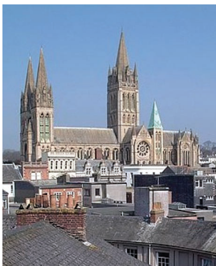
Roof top view
