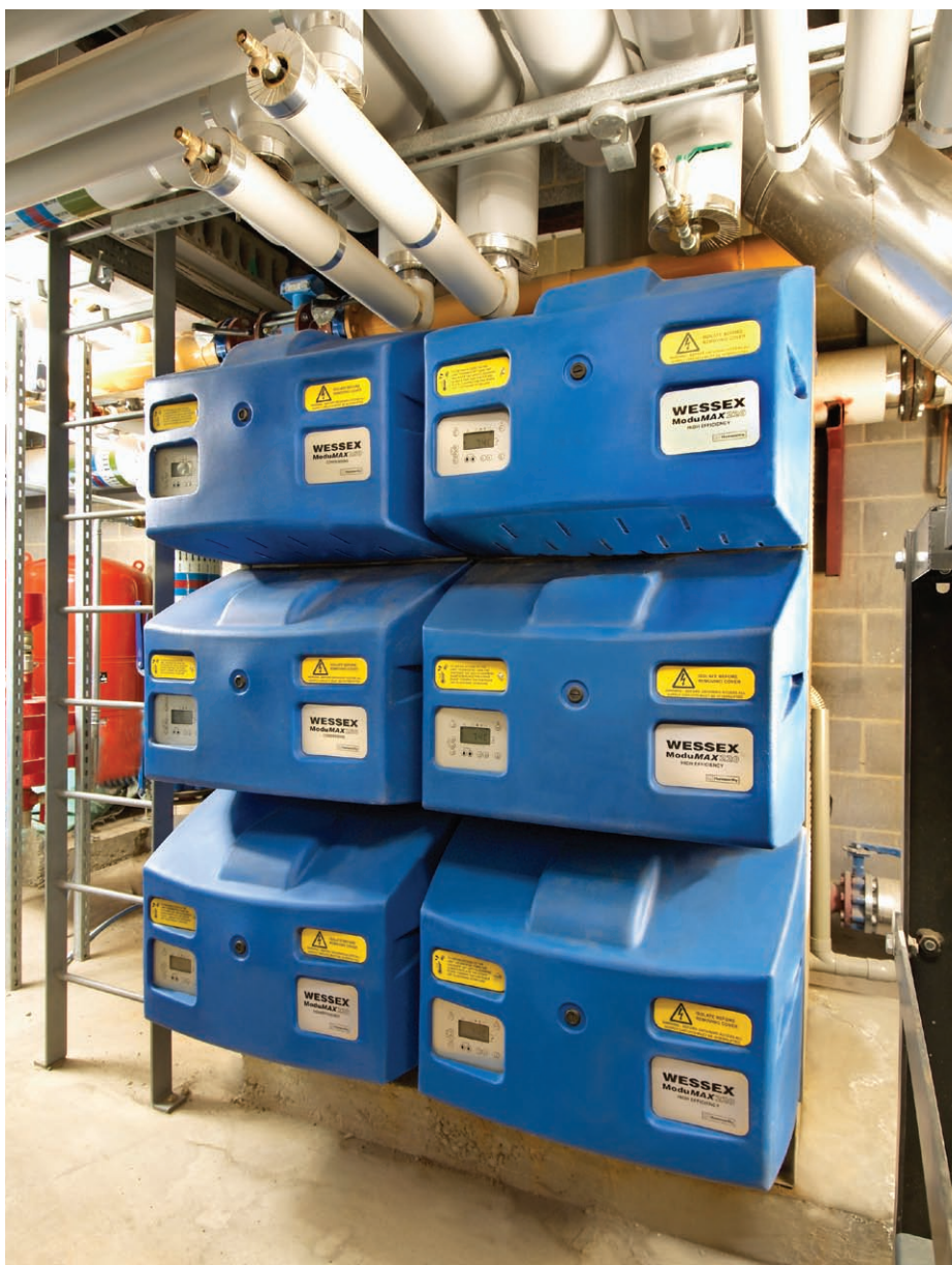
Wessex ModuMax boilers available in high efficiency condensing and non condensing models
