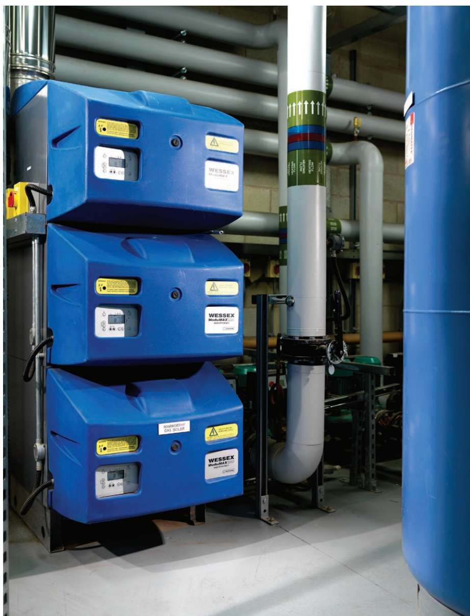
The compact Wessex ModuMax modular boilers
