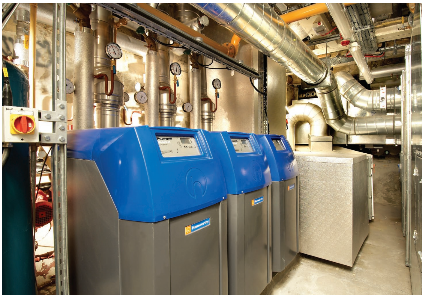
Hamworthy Purewell VariHeat boilers for multiple boiler installations
