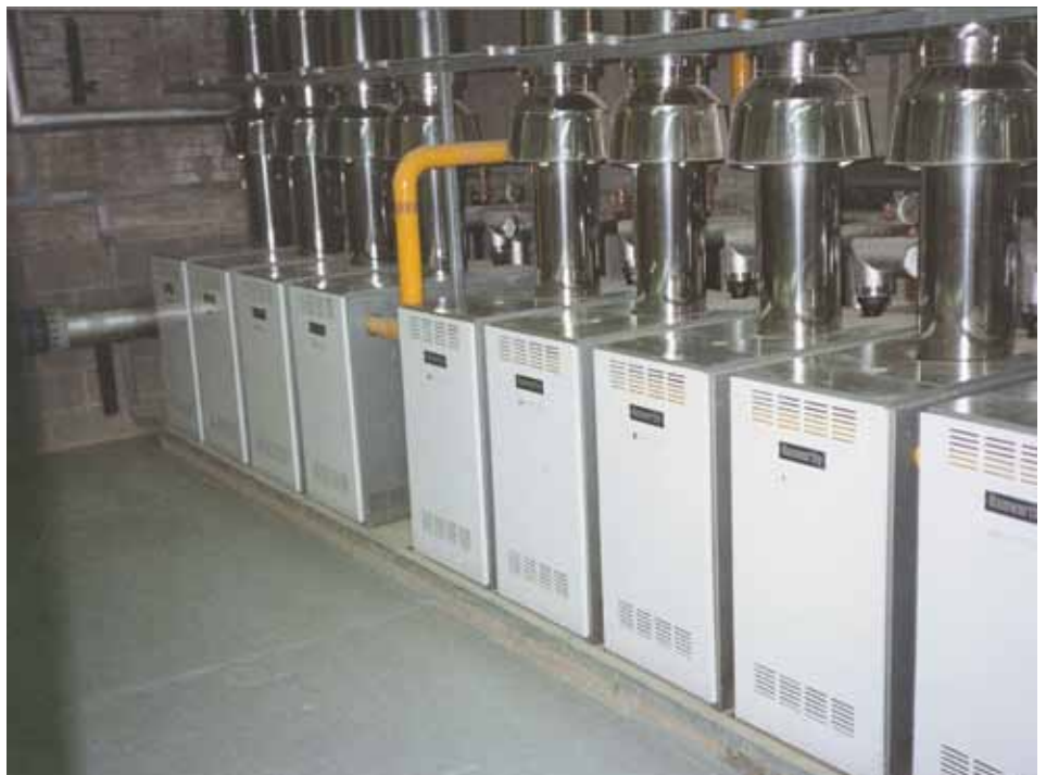
Cast iron atmospheric on/off modular boilers.
