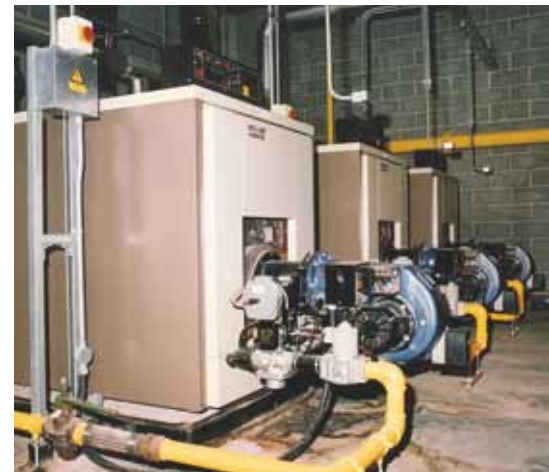
Old sectional cast iron boilers.
