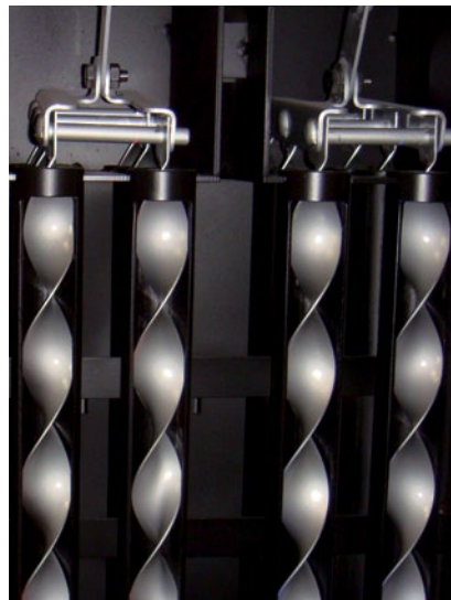
Helical turbulators in the heat exchanger
