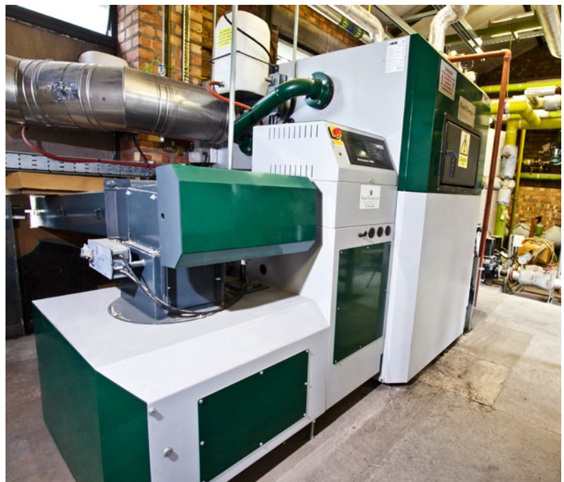
BioMatic boiler in a typical installation.
