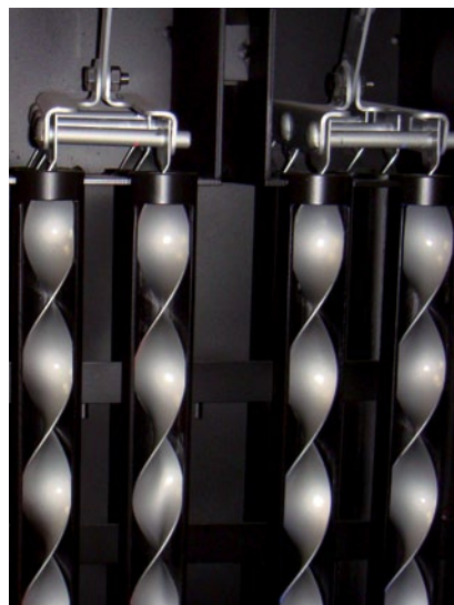
Helical turbulators
