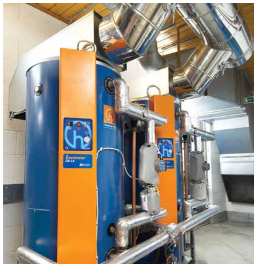
Horizontal flue off-take for simplifying the flue system when replacing old water heaters.
