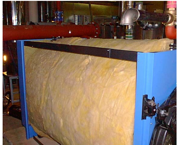
Picture 6: Side Rail attachment.
